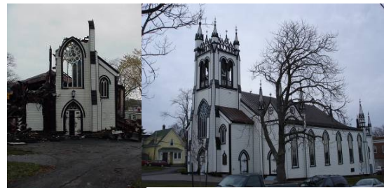
St. Johns Church Fire Damage/Restoration
